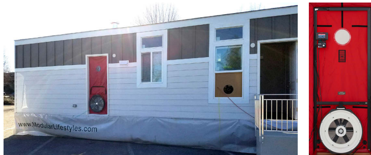
(Right) A Blower Door test was done after the house left the factory and before it was delivered to the site.
